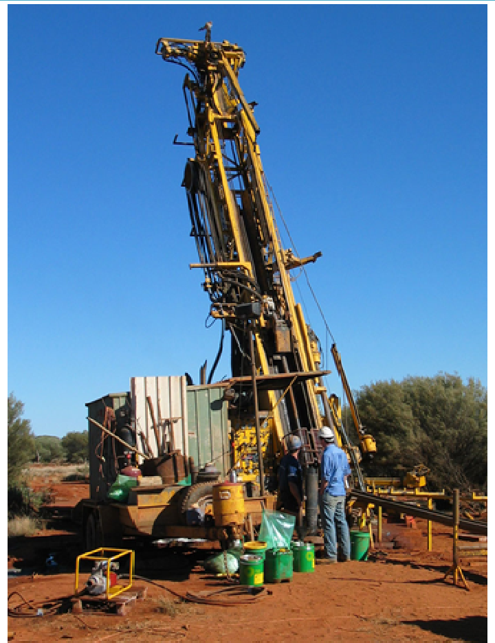
Example of drilling operations
